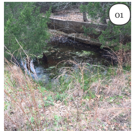
Standing water at existing foundation
